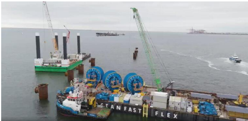
Installation of the PLEM at Wilhelmshaven 2 LNG Terminal; Source: Geocean
